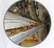
Backed up water from clogged gutters can make its way through your roof and cause cracking, leaking and other serious interior damage.
