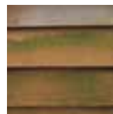
Mold on real cedar clapboard
